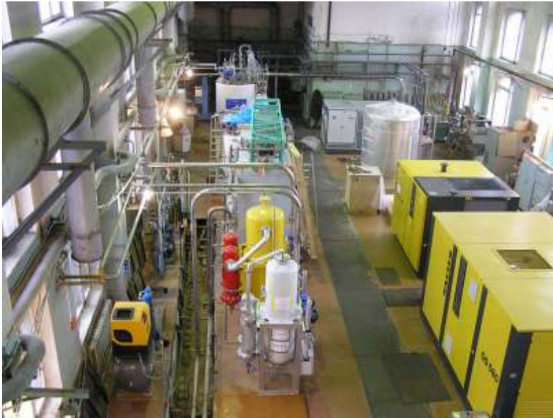
Hall of the cryogenic equipment
