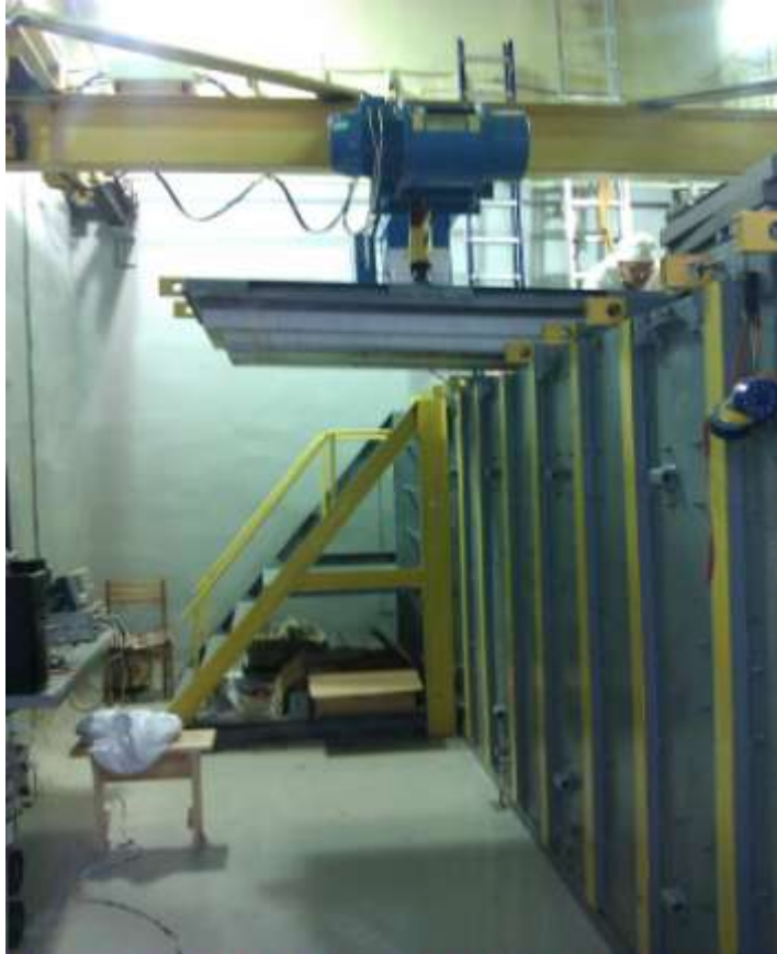
Passive shielding of 60 tons
