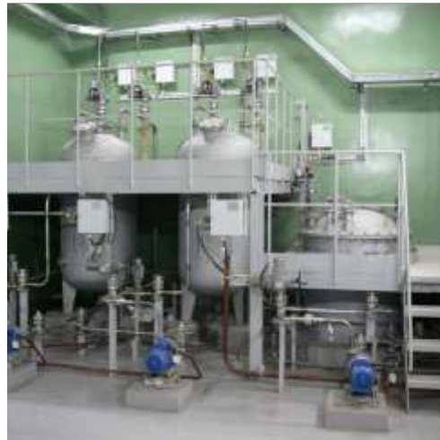
Building 122 - Emergency storage of liquid radioactive waste
