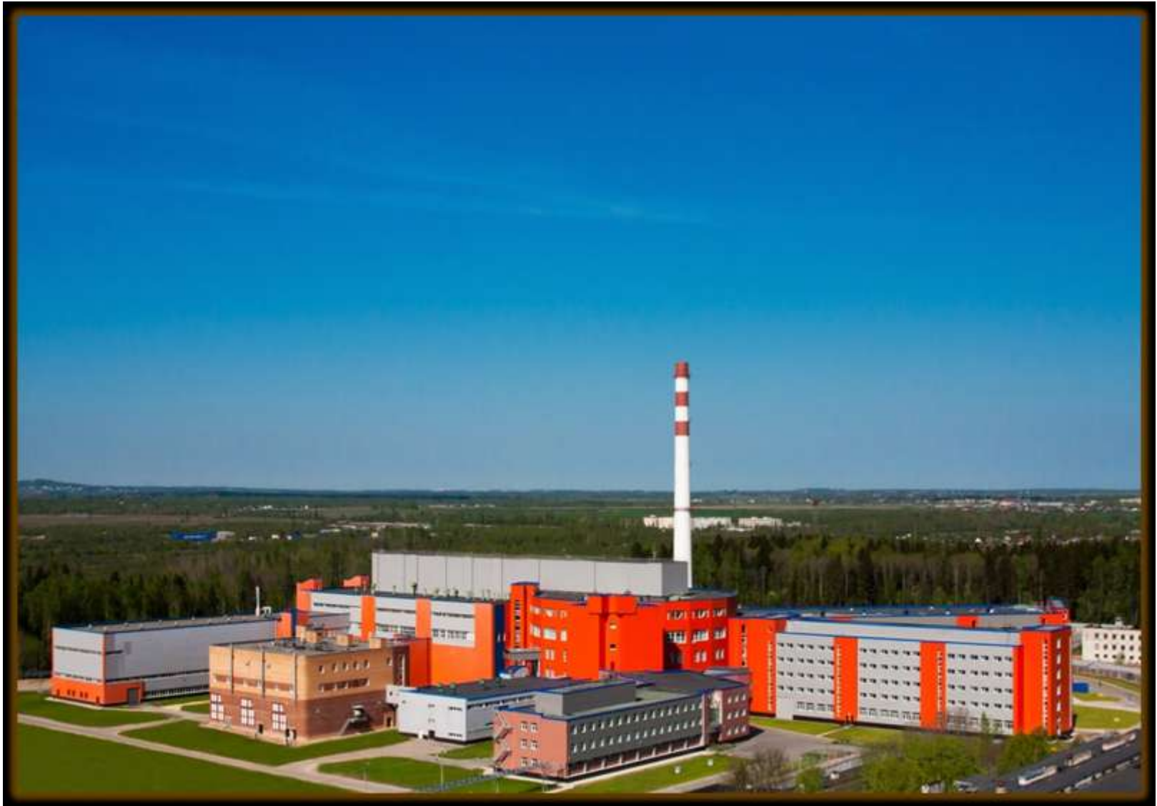
Central part of the reactor complex PIK (2014)
