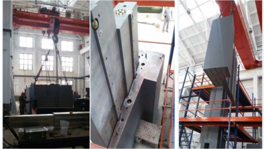
Neutron Shutter installation
