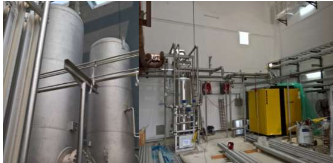
Cryogenic equipment installation
