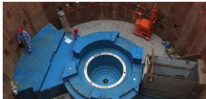
site installation of fixed shielding
