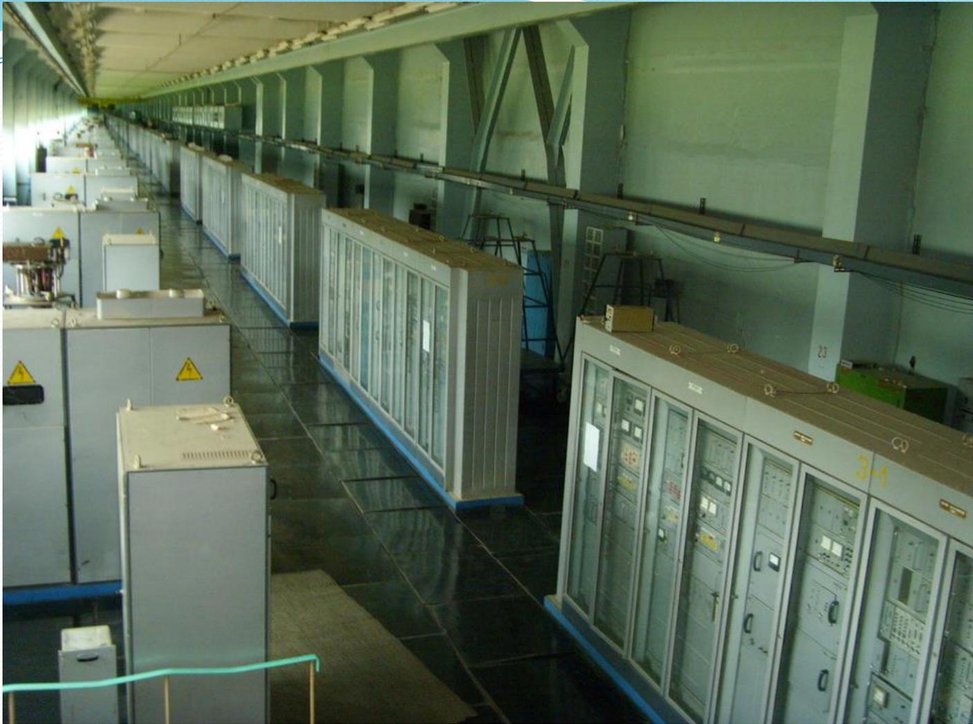
Gallery contains 33 channels of 991 MHz RF amplifiers, length is 360 meters.
