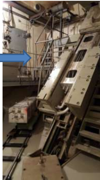
Rail track and safety shield
