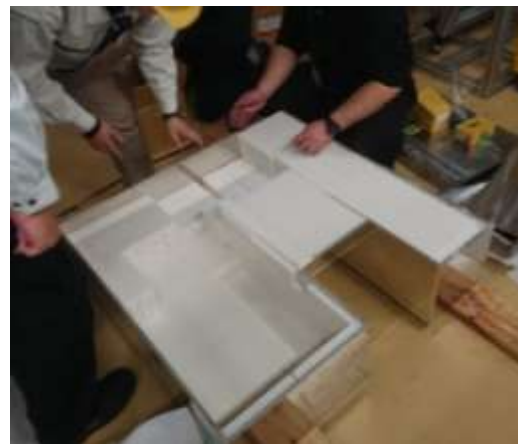
Making customized shielding block
