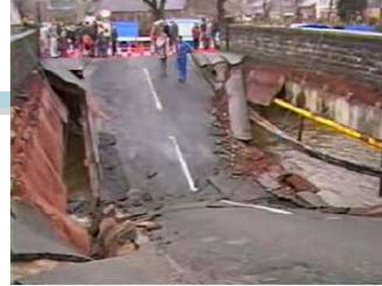
Collapse of the Ynys-y-Gwas brg. (UK, 1985)
