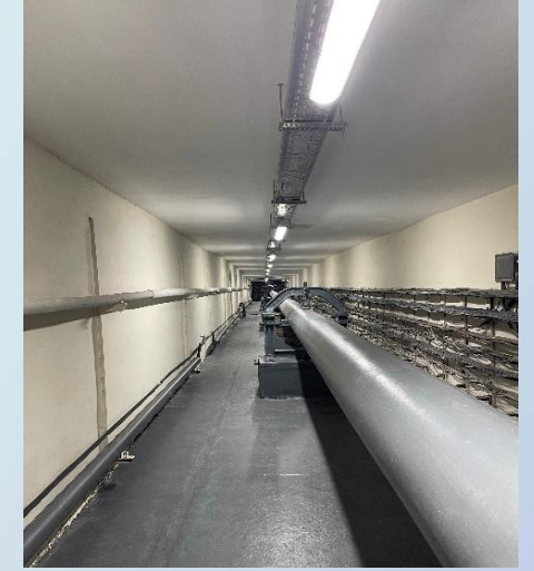
Experimental hall at IREN facility
