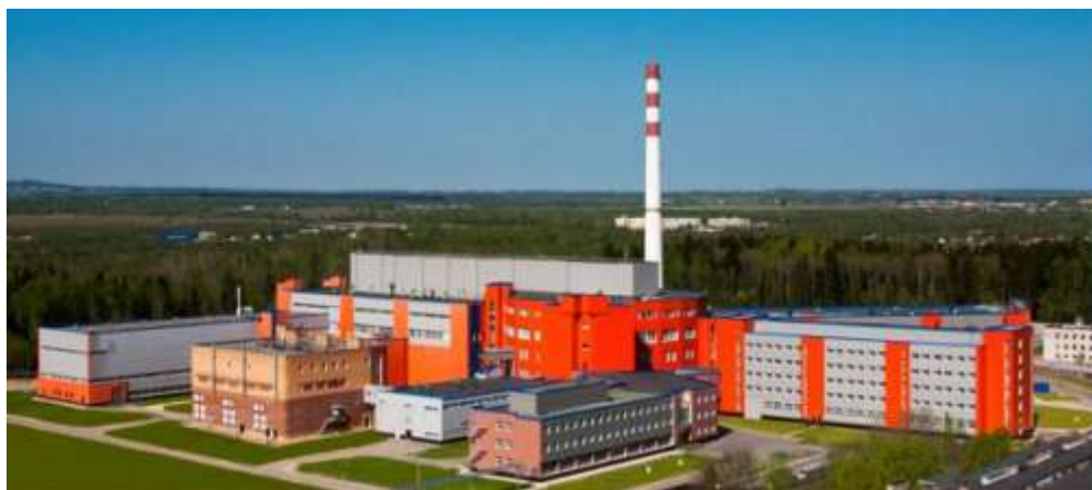
Fig.1. General view of the Reactor Complex PIK .
